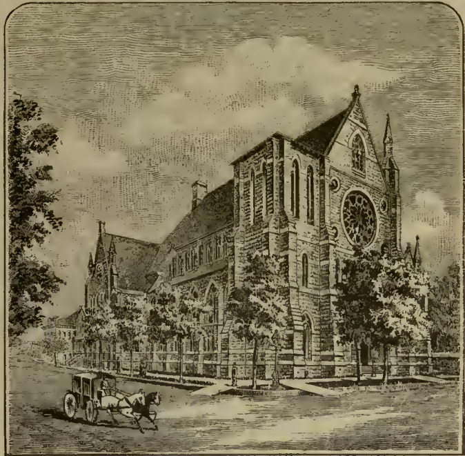
SECOND PRESBYTERIAN CHURCH; BEFORE COMPLETION OF STEEPLE.
